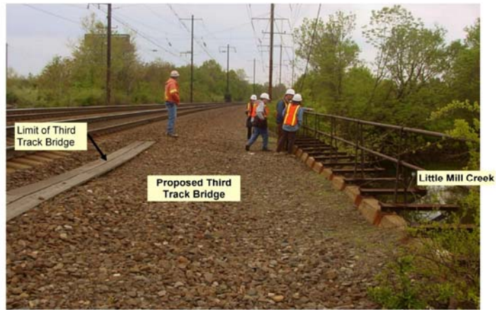
DTC - NEC Commuter Rail Improvements Little Mill Creek Crossing (Looking South)
