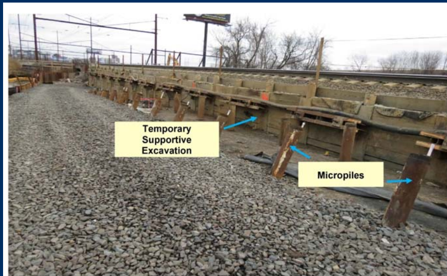
Track 2 Looking North
